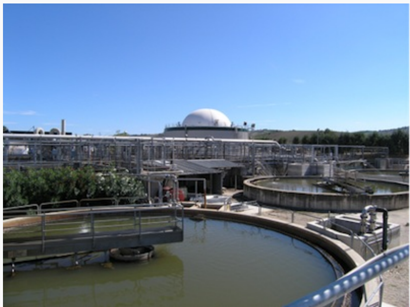
An anaerobic digester at a food processing plant in Teramo, Italy, treats poultry slaughterhouse wastewater and breeding waste to create biogas that powers a boiler and an electrical cogenerator.
